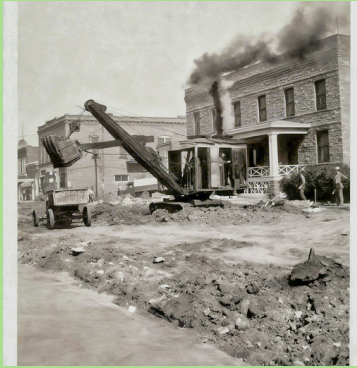
Paving Downtown Dell Rapids (c. 1929)
